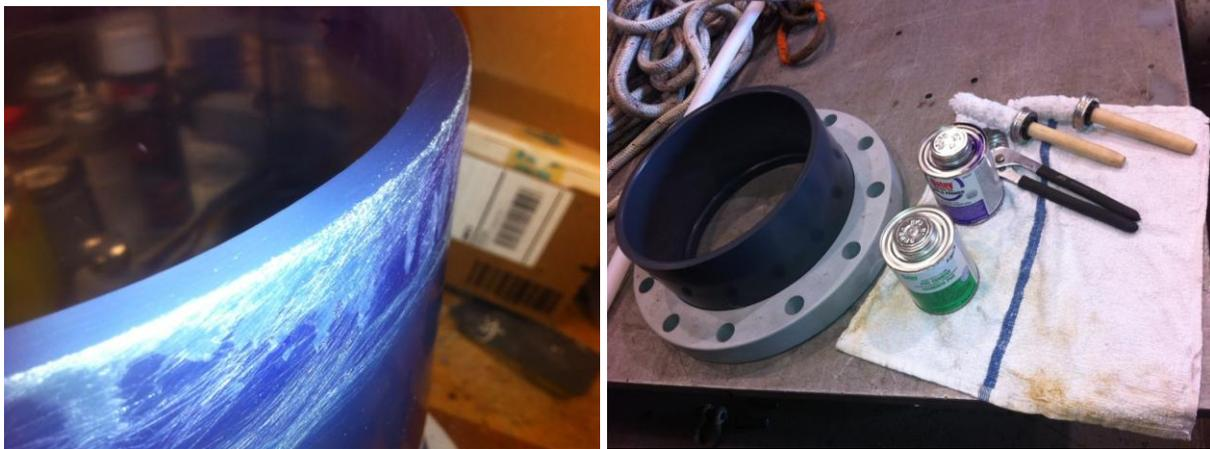
Part assembly has to be done quickly once the cement is applied so have two people ready to stand on a plate across the upper end. Following 1st image shows pipe fully engaged when assembled. A press (photo) is handy but not necessary.
