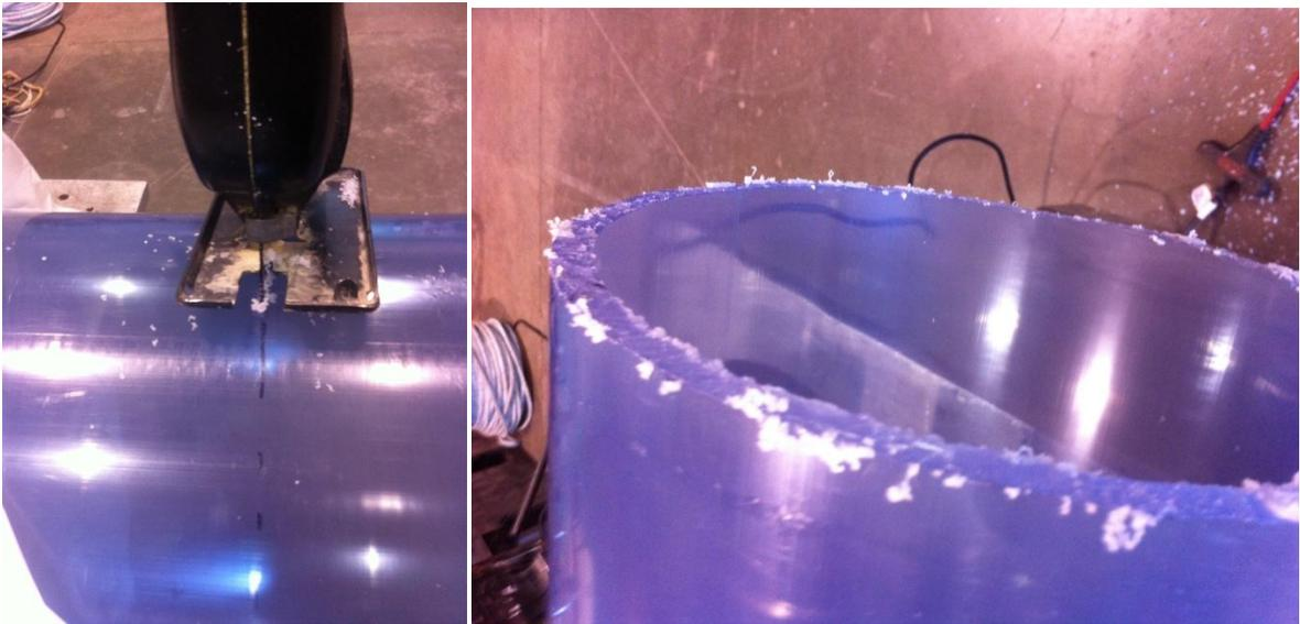
The pipe sections are cut to length square as possible and the edges beveled, sanded and cleaned.
